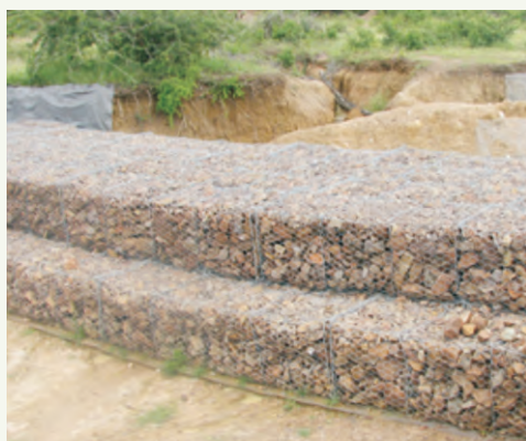
Gabions to prevent soil erosion
